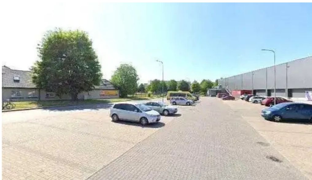
Beenergised charging station visi
