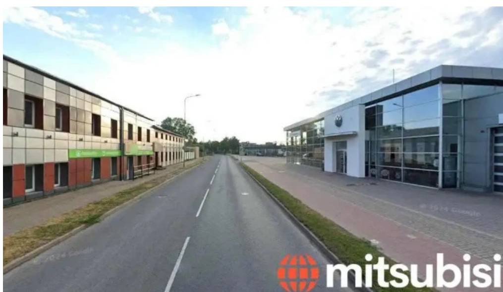
Elektrum charging station liep?ja
