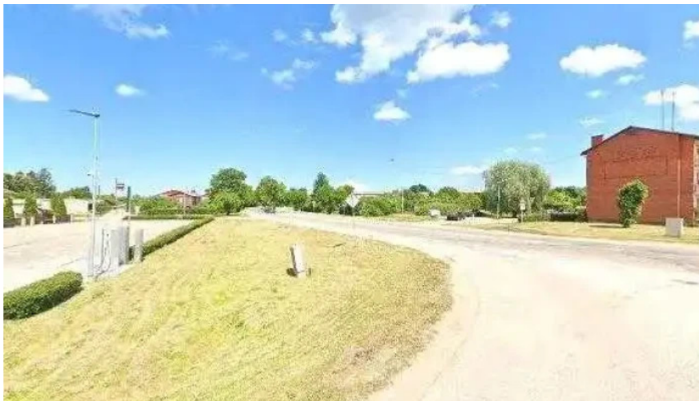
Csdd charging station visi
