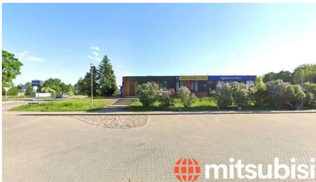
Csdd charging station aizpute
